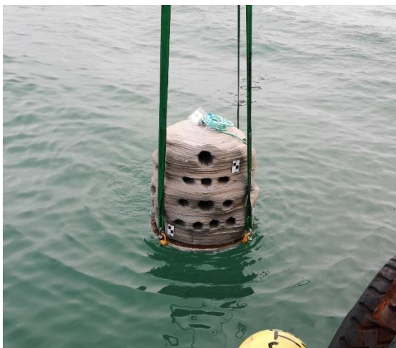
Figure 6: Deployment of 3D-printed reef in Poole Bay, UK (credit: 3DPARE)
